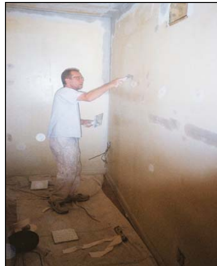
Working on the basement walls
